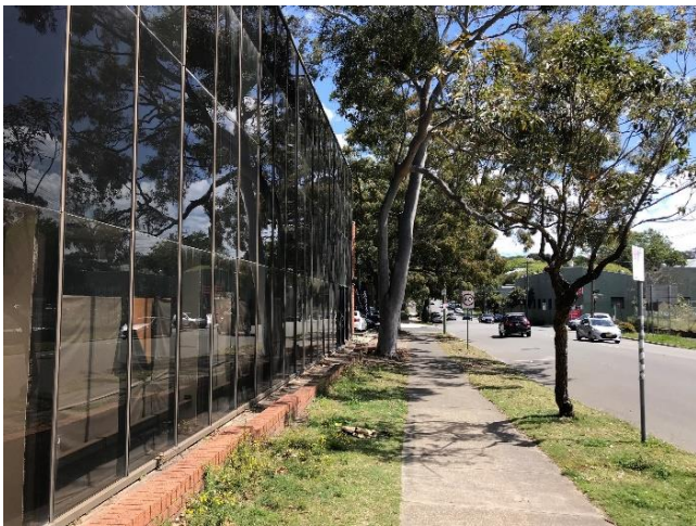
Figure 21 View to the west along McEvoy Street within the frontage of the site
